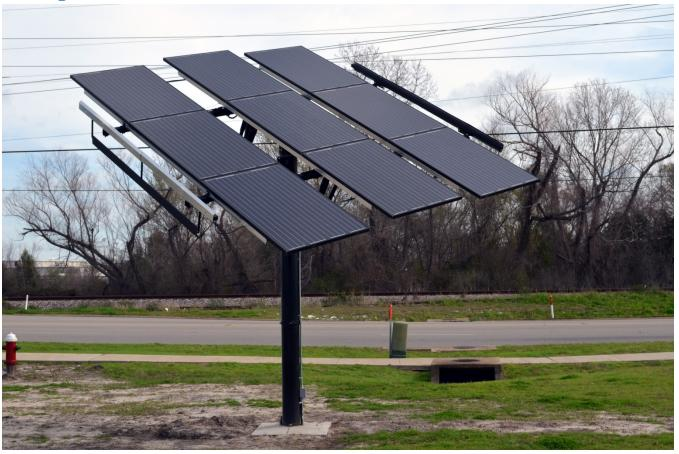
**Description** – 20kW solar photovoltaic system; 15kW of the panels were rooftop-mounted. The remaining 5kW of the panels were mounted onto custom-made monopole mounts near the entrance to the facility for advertising as well as power production purposes. The pole-mounted panels track the sun throughout the day.
