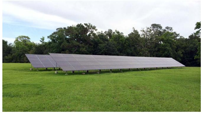
**Description** – 42kW solar photovoltaic system with 18kW emergency battery backup system and 18kWh of energy storage. The solar panels were installed on the ground using racking hardware by ProSolar. The emergency backup power system powers the entire building.
