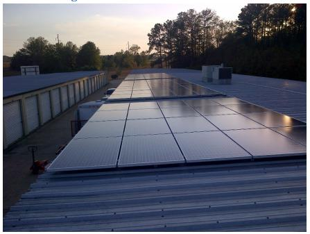
**Description** – 23kW solar photovoltaic system – The panels were mounted on the conditioned storage building rooftop. The system produces power primarily to offset the energy used by the air conditioning systems in the climate-controlled storage units.
