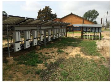
**Description** – 115kW solar photovoltaic system - 80% of the panels were installed on the ground using racking hardware made by ProSolar. The remaining 20% of the panels were mounted on the rooftops of three separate buildings. In the Ranger Station building, we also installed an 18kW emergency battery backup system and 34kWh of energy storage. The emergency backup power system keeps the food storage refrigerators, lights, computers, and cash registers going during grid power outages.
