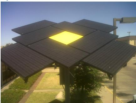
**Description** – 3kW solar photovoltaic system mounted onto custom-made monopole mounts near the entrance to the facility. The primary purpose of this system is to promote solar energy and provide visible evidence for utility customers that BTU invests in solar power. The pole-mounted panels track the sun throughout the day and throughout the year (dual-axis tracking).
