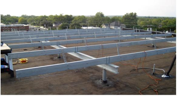
**Description** – 10kW solar photovoltaic system – The panels were mounted onto a flat rooftop in the historical district of downtown Bryan, TX. Due to the age, historical significance, and construction of the building, we designed custom framework to tie into the building main beams and load-bearing columns rather than the traditional method of loading the roof structure itself.
